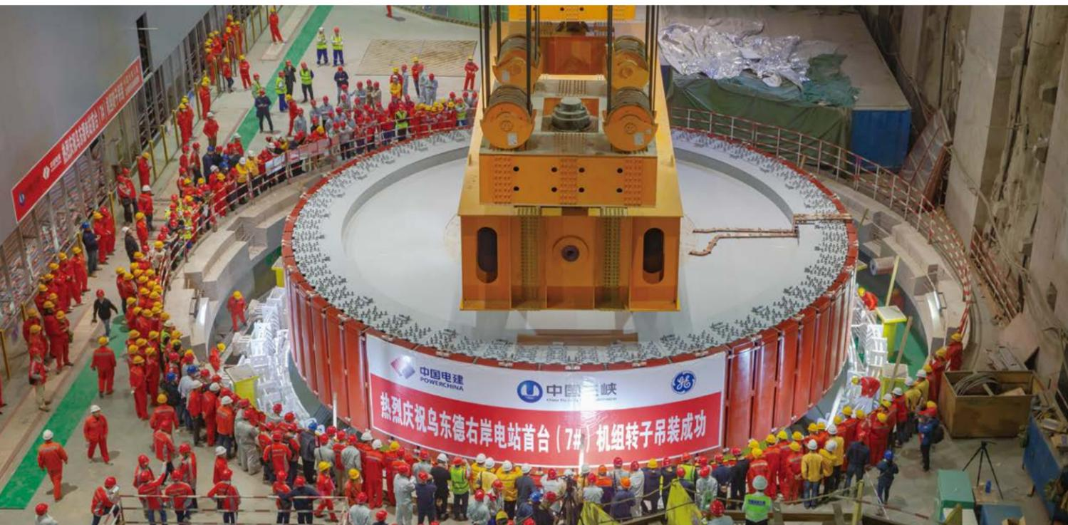
Workers hoist the rotor of the first power unit (No. 7) on the right bank of the Wudongde Hydropower Station
