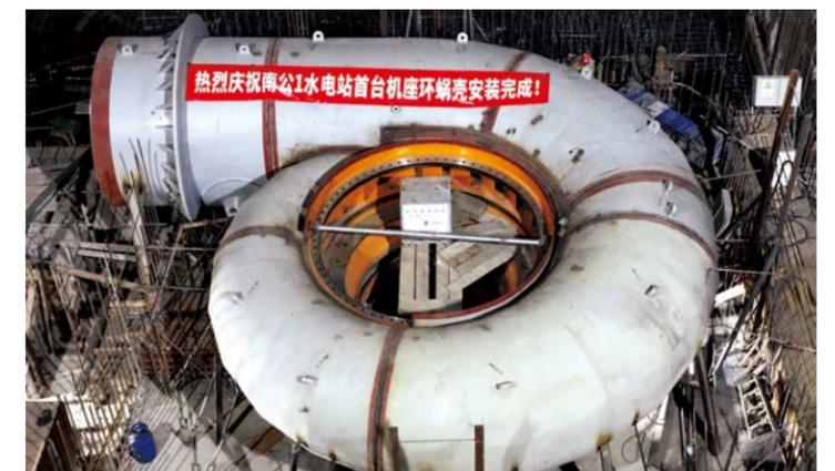
Nam Lik 2 Hydropower Station in Laos installs the turbine case on the seat ring of its first power unit
