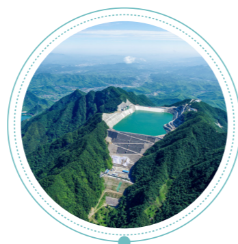
Changlongshan Pumped Storage Power Station
