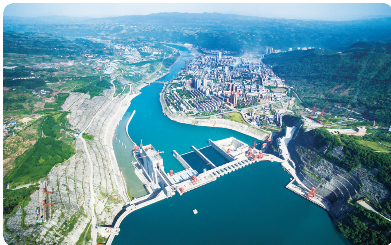
Xiangjiaba Hydropower Station
