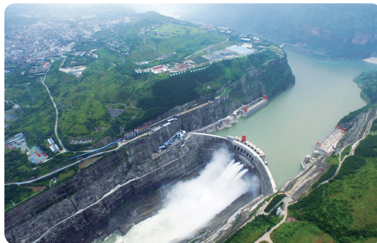
Xiluodu Hydropower Station
