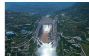
Xiluodu Hydropower Station Project kicked off construction
