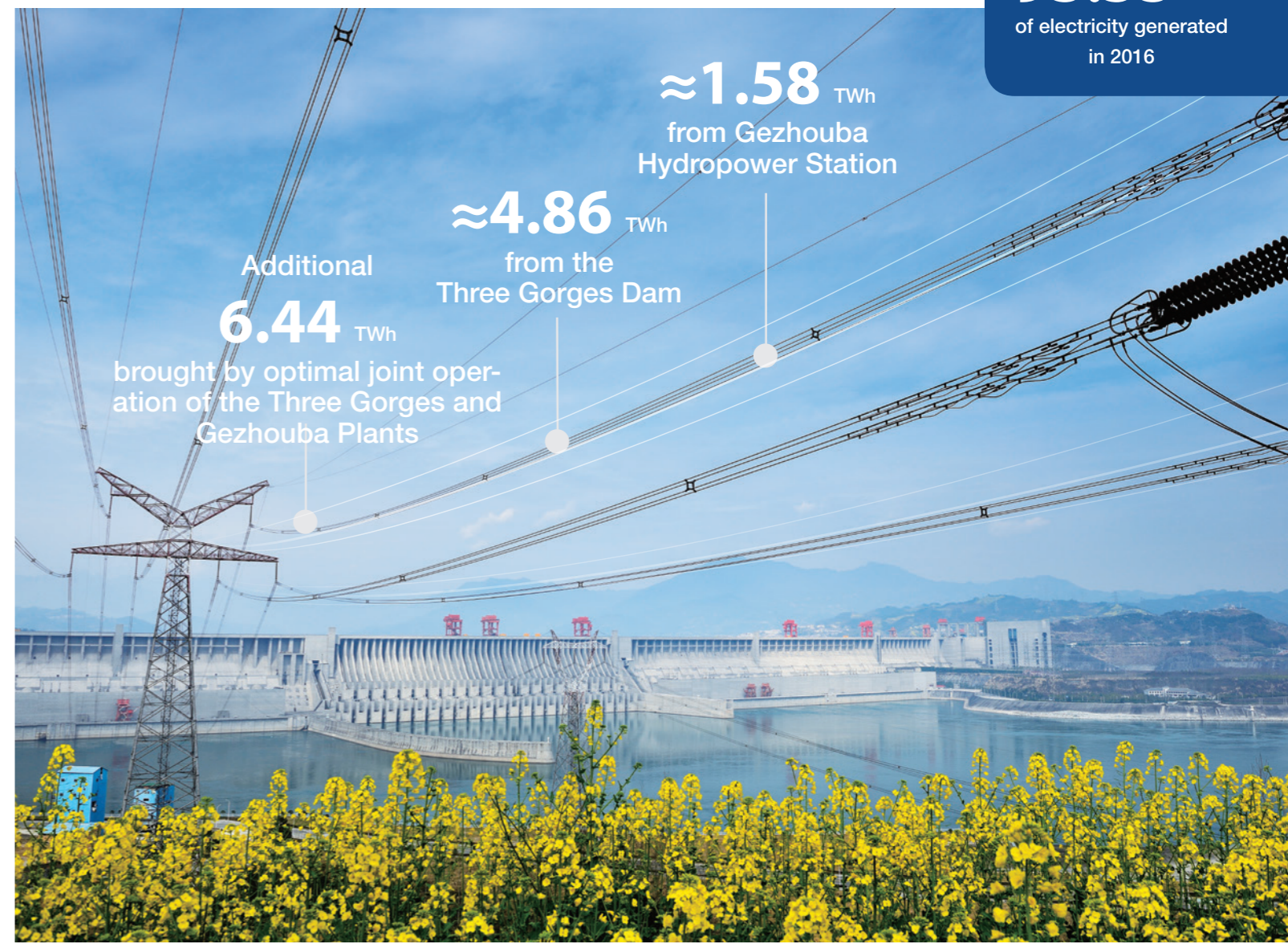
Power Transmission Lines of the Three Gorges Power Station
