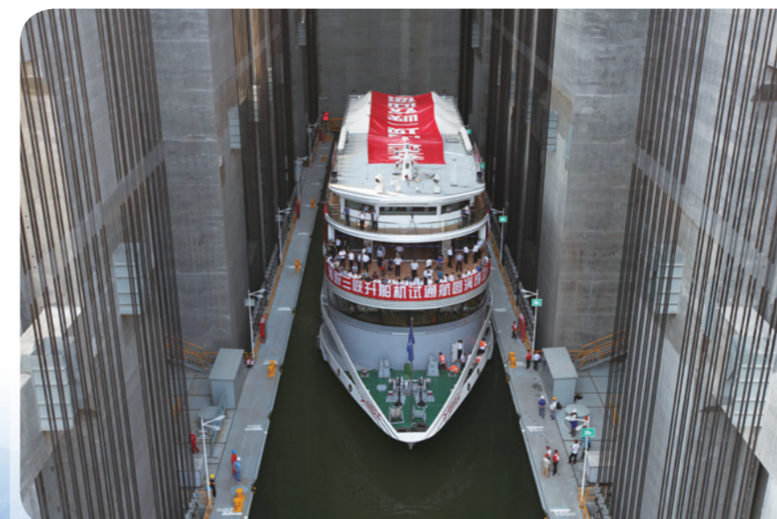
On the afternoon of September 18, the "TG 9" passenger liner was shipping into the ship lift chamber, which signaled the beginning of trial operation of the ship lift and the completion of the project construction.
