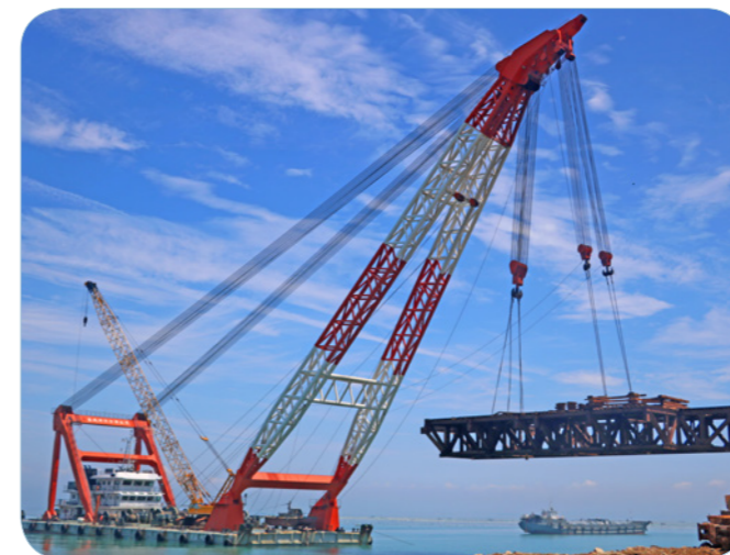
Pilot offshore wind farm under construction at Xinghua Bay, Fujian.
