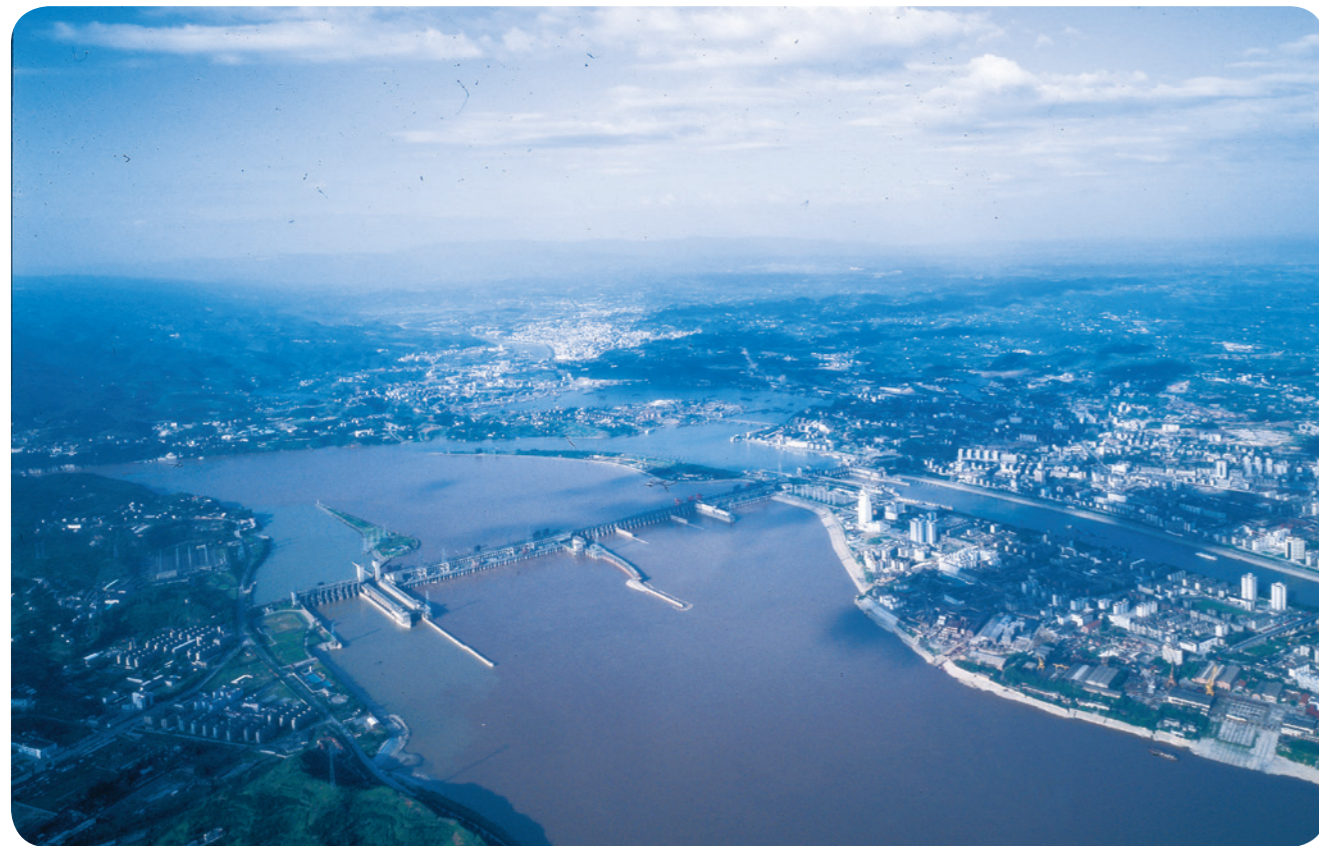
Gezhouba Hydropower Station
