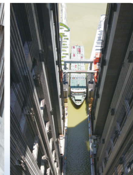
Commercial vehicle carrier into the ship lift chamber
