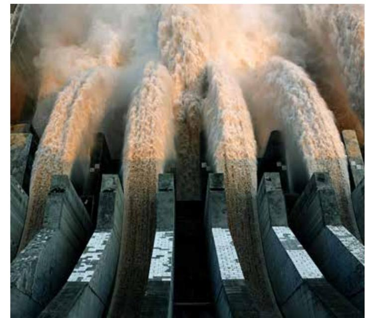
As the Yangtze River No. 1 flood in 2018 passes through the TGP reservoir, the Three Gorges Hydropower Station opens up deep holes to discharge the flood waters
