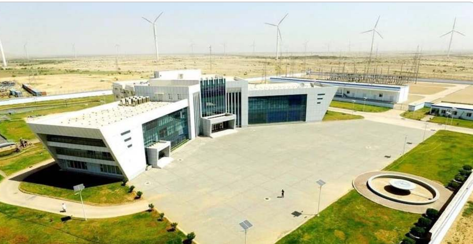
Panoramic View of Three Gorges Wind Farm Projects and Office Complex
