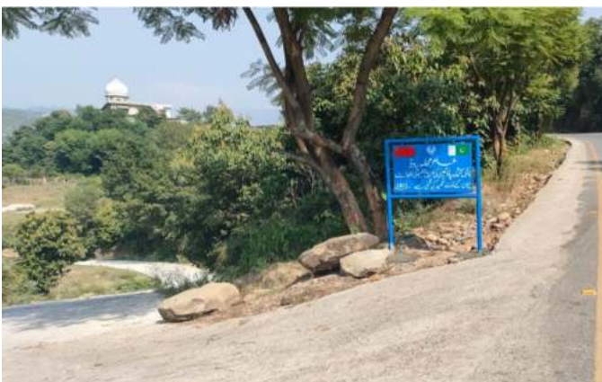
Newly Constructed Access Road in AJK
