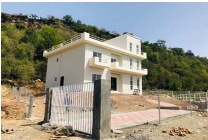
Newly Constructed Rest house in Hollar village, AJK
