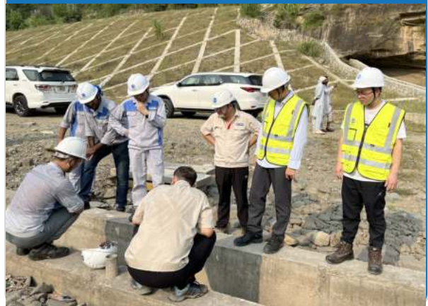
Safety Inspection at the site of Karot HPP
