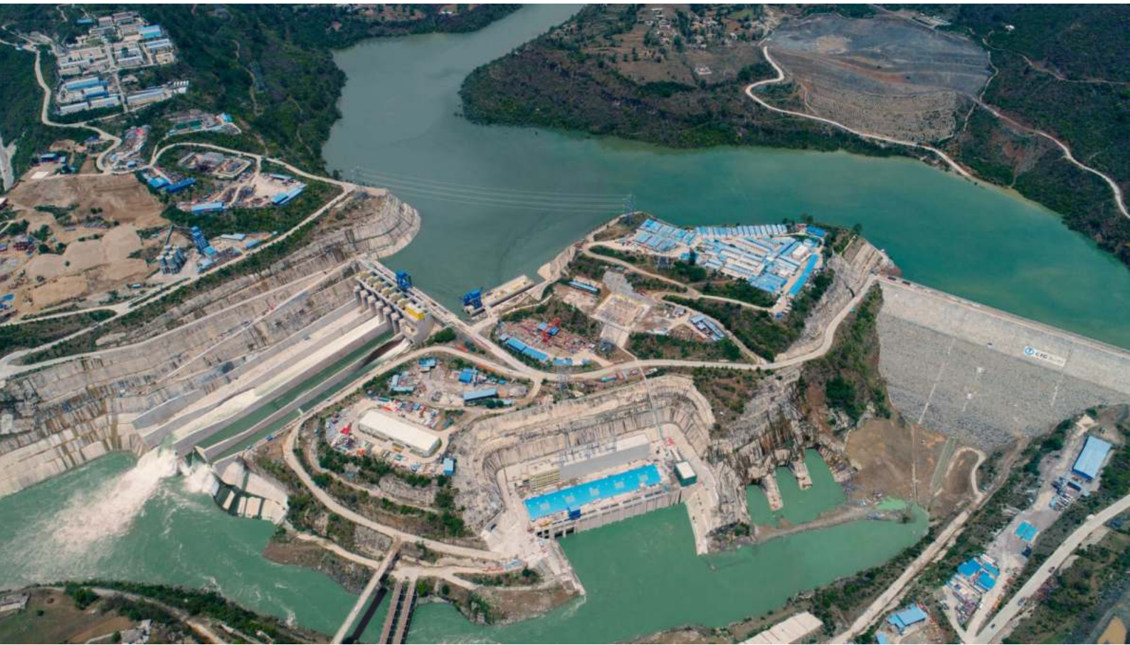
Panoramic View of 720MW Karot Hydropower Project, Pakistan
