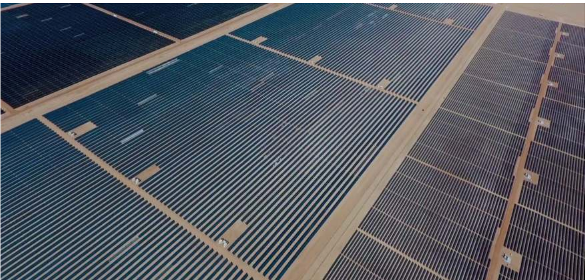
Panoramic View of Aten and Horus Solar Energy S.A.E. Projects
