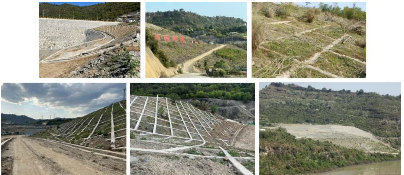
Erosion control practice and slope protection at Karot HPP
