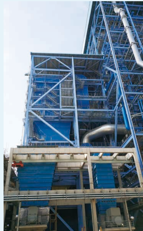
Flue gas denitrification device for Phase III of the project
