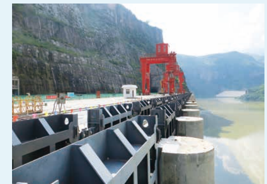
Stratified water intake through stoplogs gate in Xiluodu
