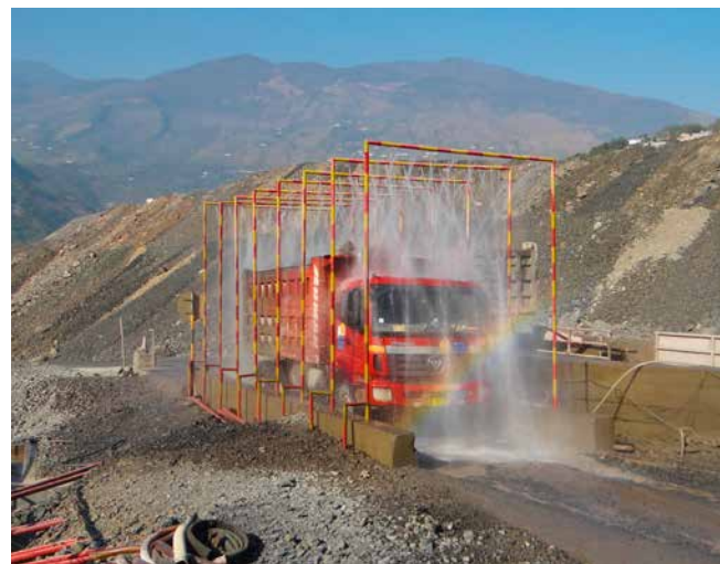
Slag truck washing and rinsing system of Haizigou waste slag yard in Baihetan Hydropower Station
