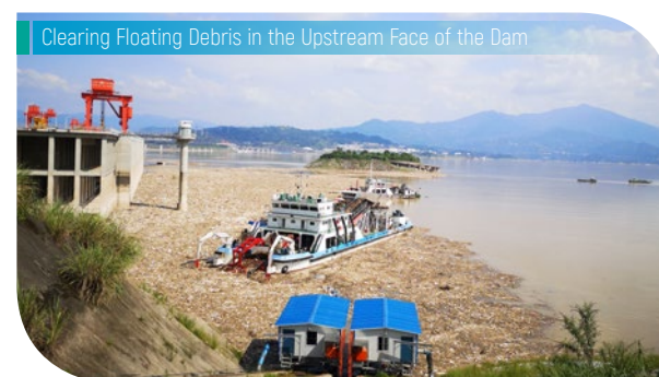
Clearing Floating Debris in the Upstream Face of the Dam
