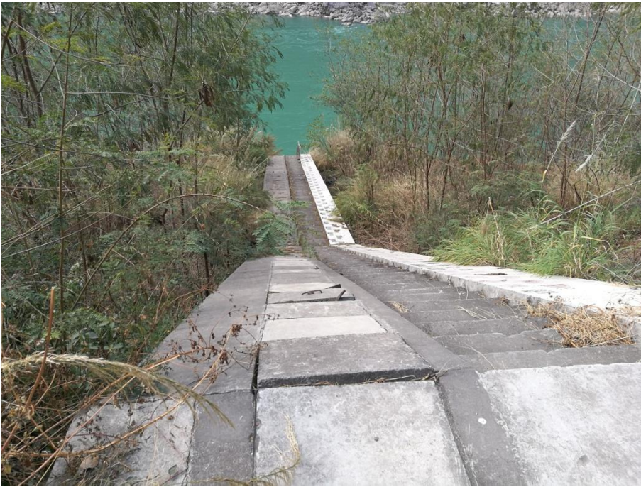
癞子沟弃渣场浆砌石排水沟、浆砌石急流槽
