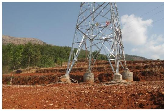
A photograph of a steel lattice tower base under construction. The ground is reddish-brown soil with concrete foundation pads. The tower structure is partially visible.  |
