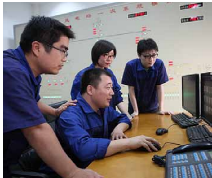
响水风场升压站中控室进行远程监控
