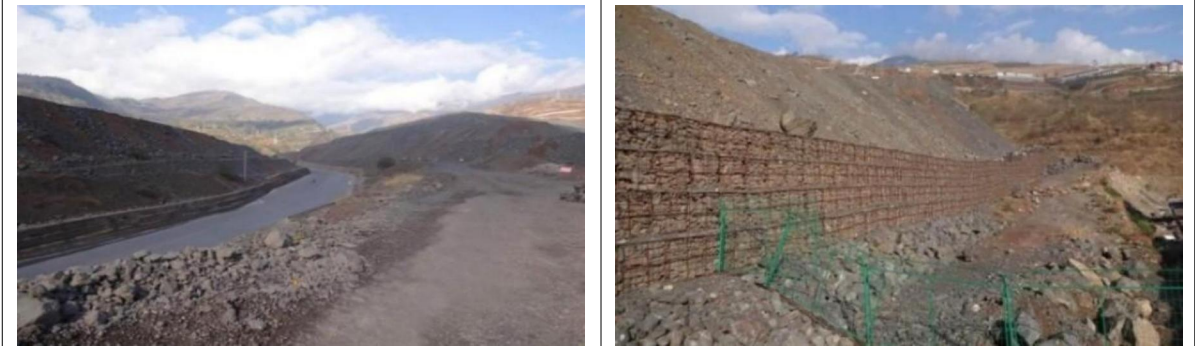
矮子沟弃渣场坡脚挡墙
